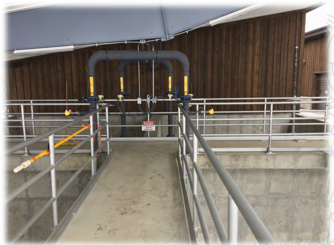
Aerobic Digesters
